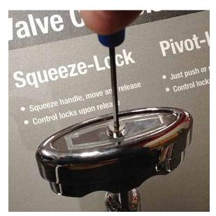
3. Using a metric allen wrench, loosen the flat head screw at the center of the handle. Be very careful while removing the handle so as not to lose the springs that load the handle.
